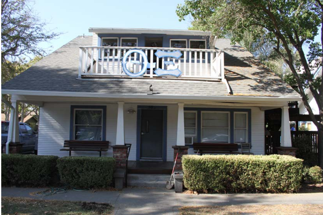
FIGURE 15: Current view of 503 1st Street with the rooftop veranda conversion.
