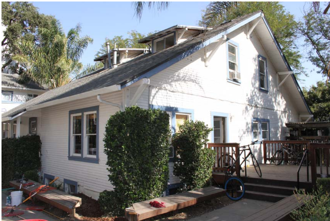
FIGURE 23: Current view looking southeast at the northwest elevation of 509 1st Street. Note the contemporary deck addition between 503 and 509 1st Street.
