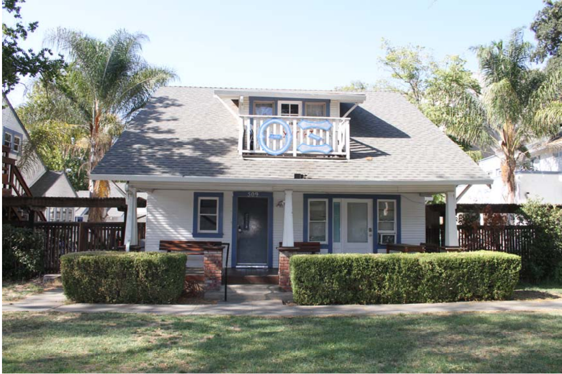
FIGURE 22: Current view looking north at the front elevation of 509 1st Street.
