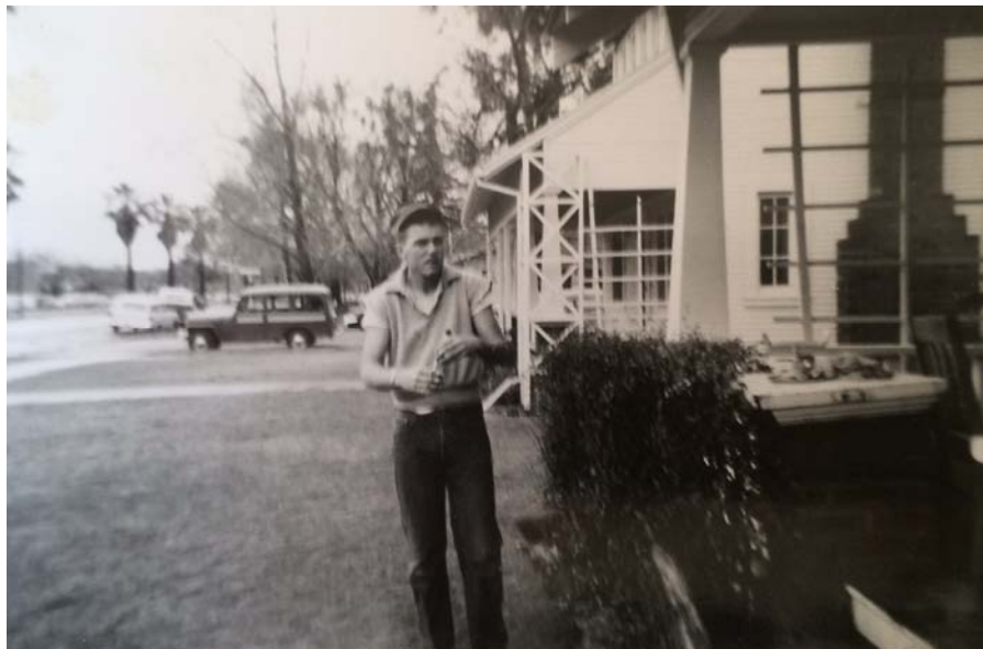
FIGURE 13: View looking west from 509 1st Street towards 503 1st Street, 1958. Note the brick chimney on the right that has since been removed on 503 1st Street (courtesy Theta Xi Fraternity).
