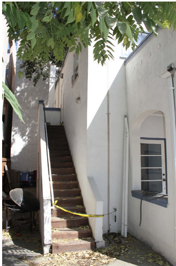
FIGURE 30: View of the north elevation of 515 1st Street. The rear stairway was apparently added when the porches were altered to provide outside access to the second story.
