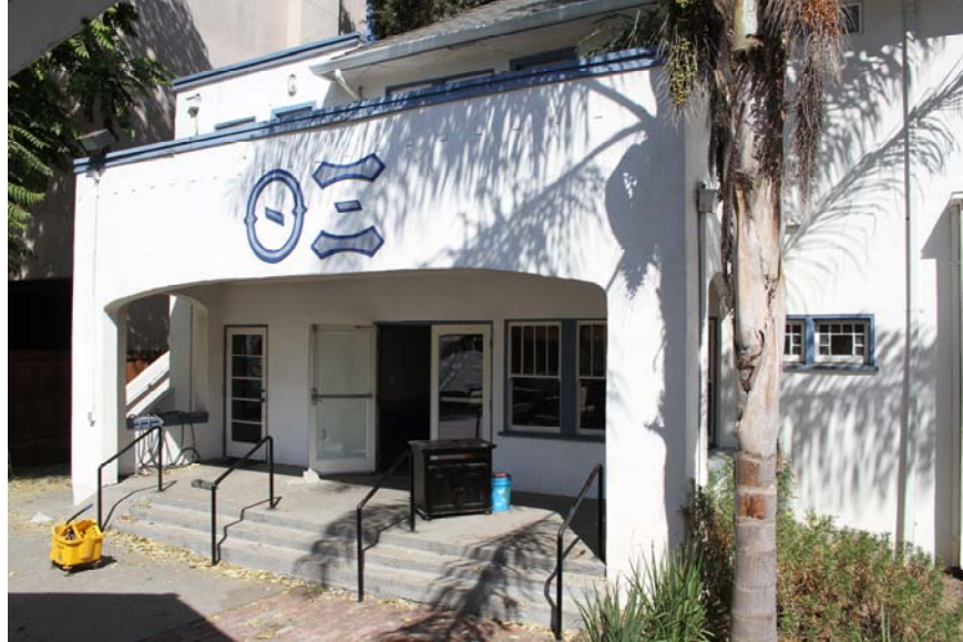
FIGURE 29: Another view of the west elevation of 515 1st Street showing the side veranda, probably remodeled the same time the front porch was reconstructed.
