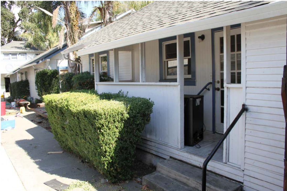
FIGURE 18: View looking east at the rear of 503 1st Street.
