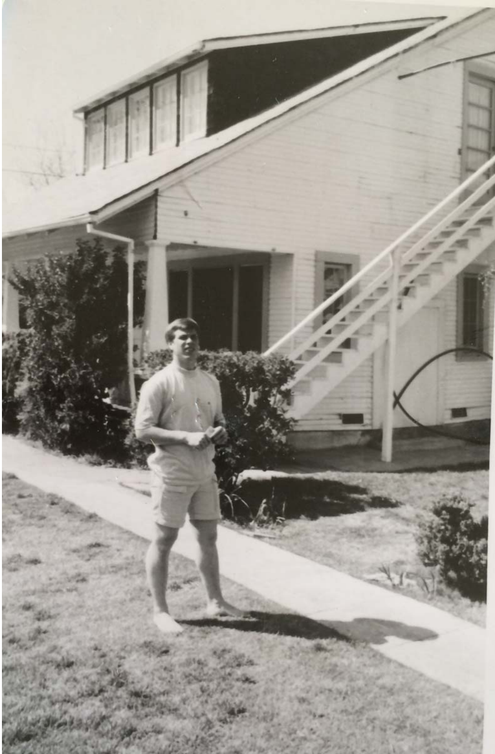
FIGURE 14: View looking west towards 503 1st Street in the 1980s depicting the added side entrance exterior stairway after opening the attic area to create dorm rooms (courtesy Theta Xi Fraternity).
